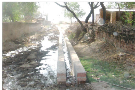
Pre-position of road work in village Ahraura
