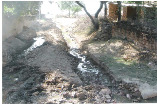
Pre-position of road work in village Ahraura
