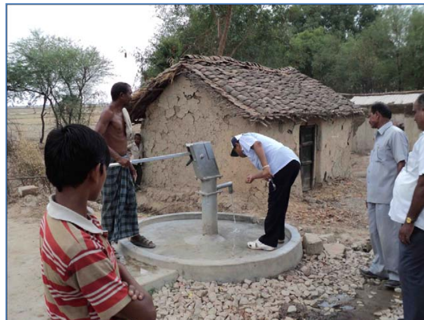
Plate 8 India Marka II Handpump in village Pathakpur
