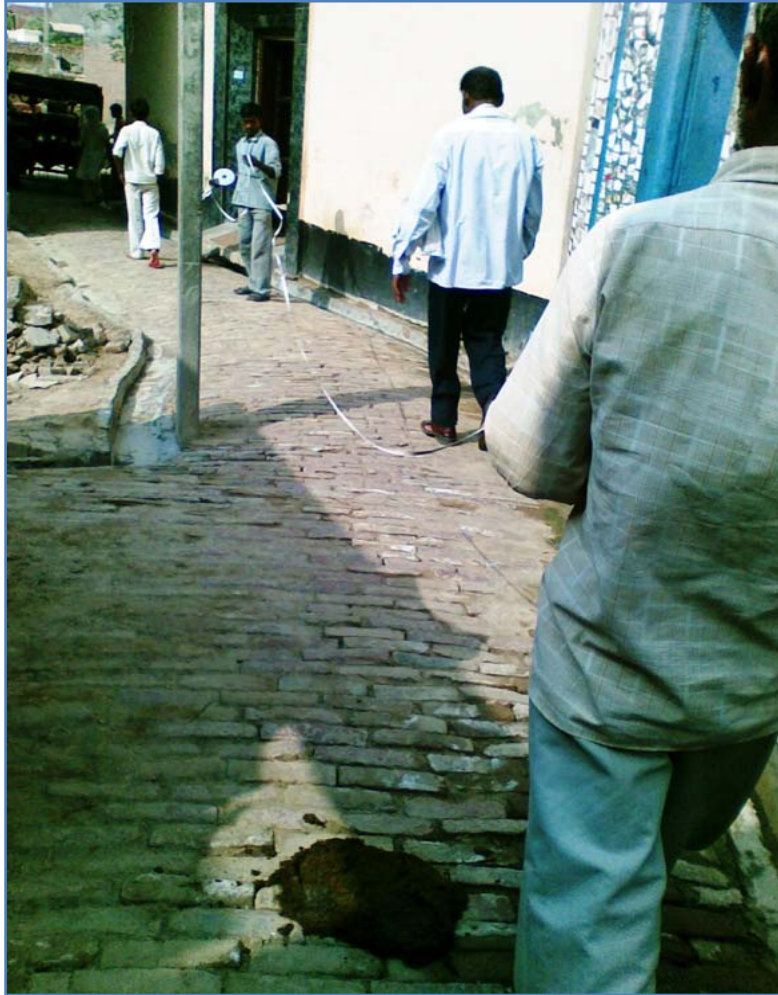
Plate 1: Repair of Kharanja in the Project Area
