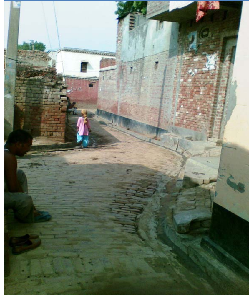
Plate 2: Repair of Kharanja & Drains in the Project Area
