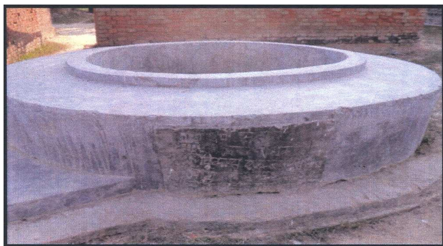
Repaire of Well No.2 Vill.-Akusi
