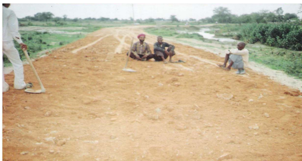
Road maintenance at Bhadokahr
