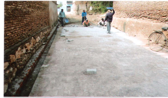
Road maintenance at Ghuraiya
