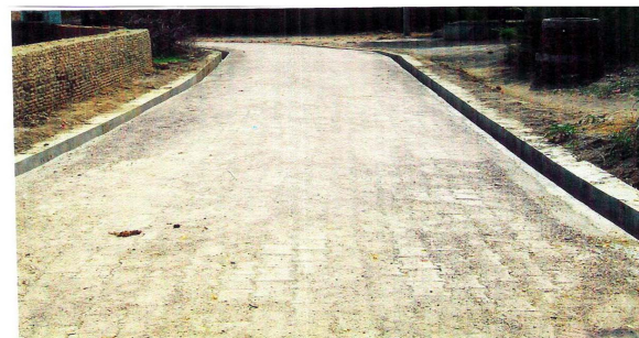
Road maintenance at Luhargaon
