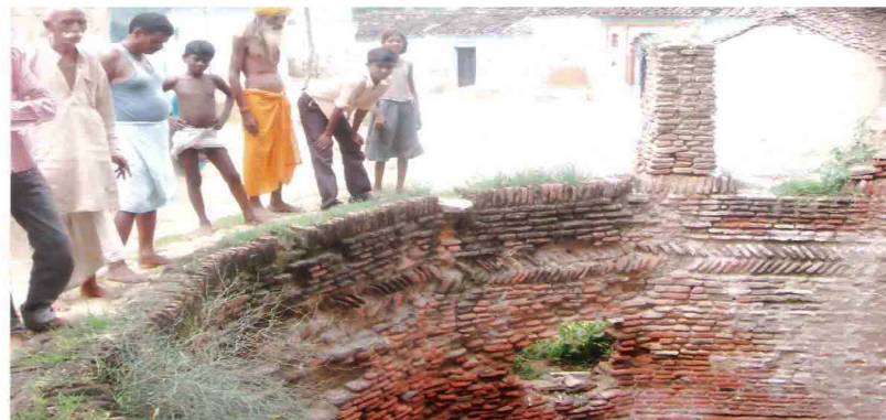
Well maintenance at Banka Pahari
