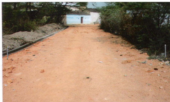
Road maintenance at Garhi Kargain
