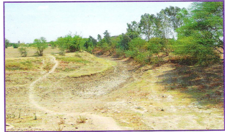
Fig. 3.2: Severe erosion in the watershed
