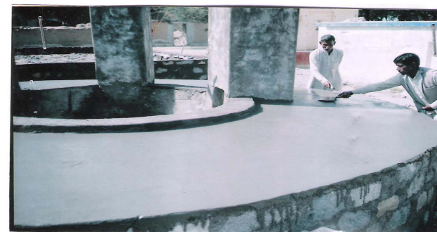
Welll maintenance at Maigaon
