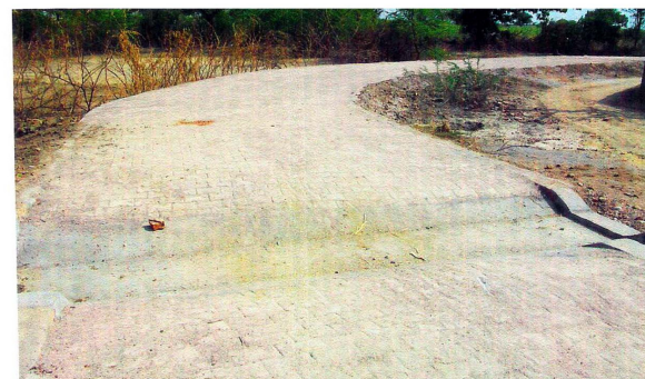
Road maintenance at Luhargaon
