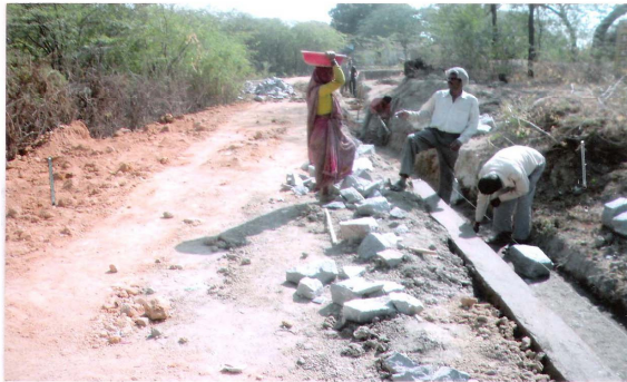
Road maintenance at Garhi Kargain
