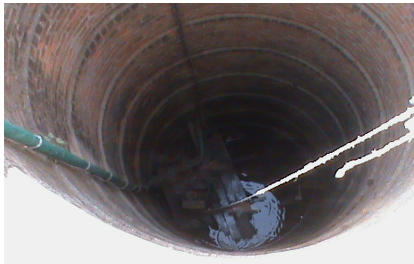
Fig. 3.6: Deep water table in open shallow dug well in the watershed
