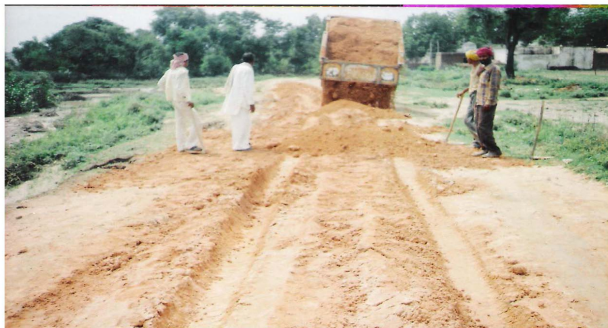
Road maintenance at Bhadokahr
