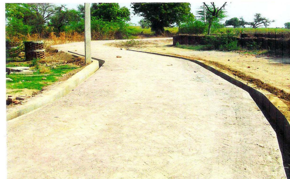
Road maintenance at Luhargaon
