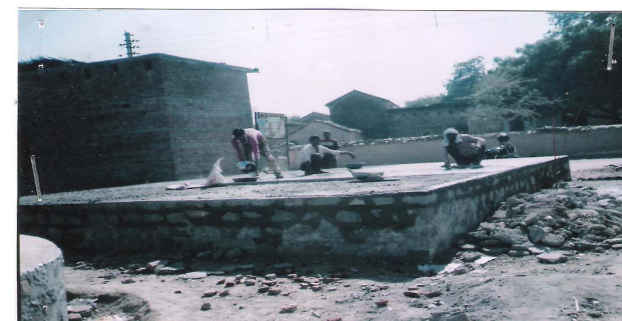
Chabootra maintenance at Maigaon
